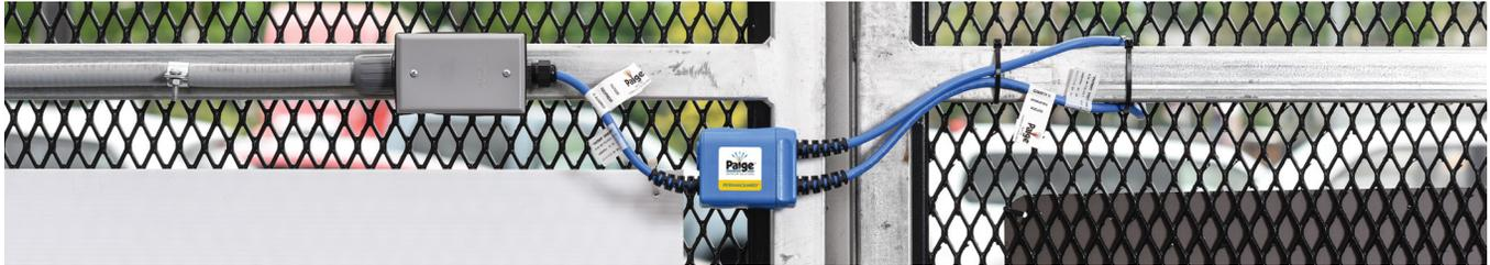
Be sure to avoid installing the cable in such a way that the cable will move back and forth against a sharp metal edge causing abrasion. We do not recommend installing in the pipe frame unless a rubber grommet or similar guard can surround the cable where it meets the metal.
